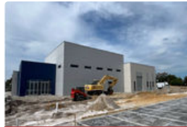
June 2024 Parking Lot Pavers Installed
