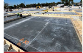
January 2024 Foundation Poured
