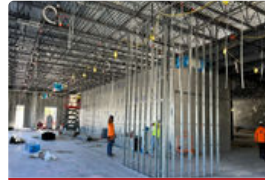
April 2024 Framing Complete
