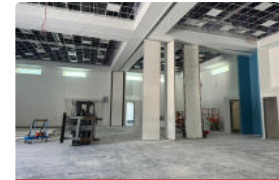
August 2024 Flooring Installed
