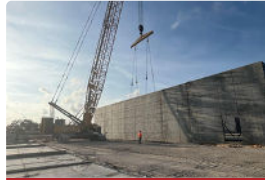
March 2024 Tilt Walls Lifted
