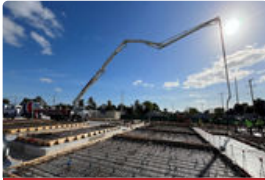
February 2024 Tilt Wall Panels Formed
