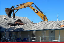
October 2023 Demolition Began
